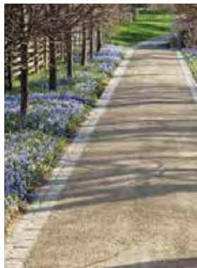
Aggregate driveway with stone edging
