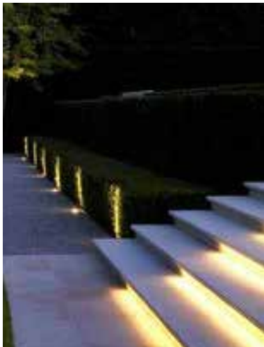
LED Strip Lighting on Entry
