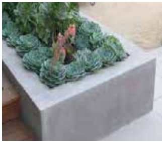
Rendered concrete block wall (retaining wall finish option)
